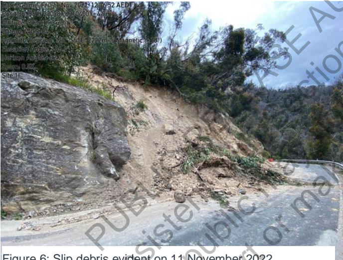
Figure 6: Slip debris evident on 11 November 2022
