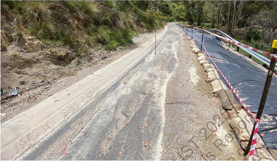
Figure 5: Loss of downslope lane - 2022
